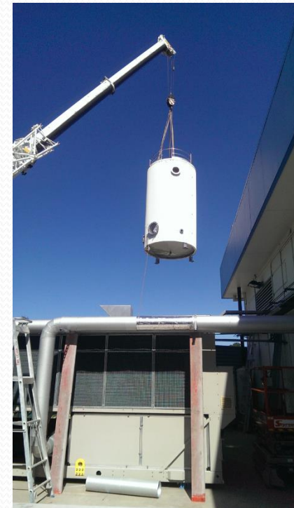
30,000L tank installation
